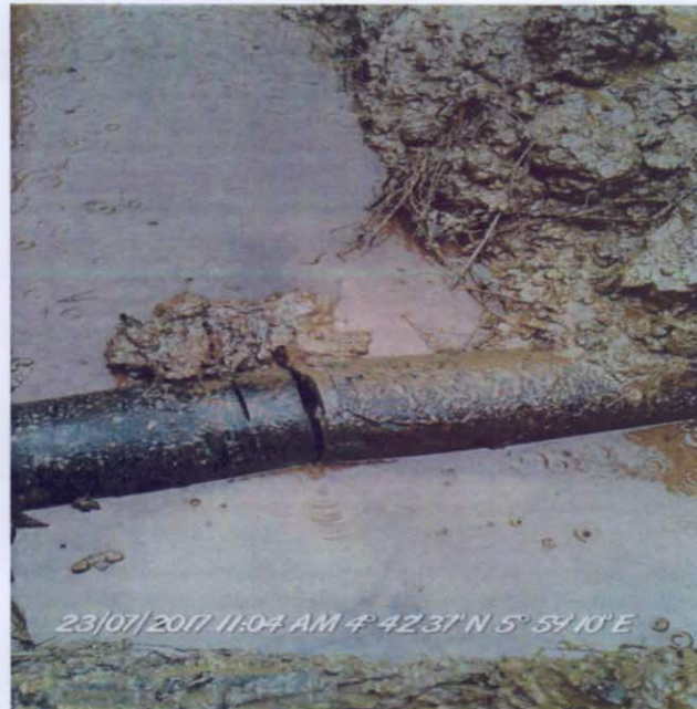
Incident Point After Excavation
